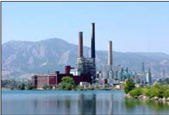
Xcel's Valmont Station near Boulder, Colorado Total Capacity 229 MW: 186 MW Coal-Fired Steam Unit plus 43 MW Gas-Fired Combustion Turbine
