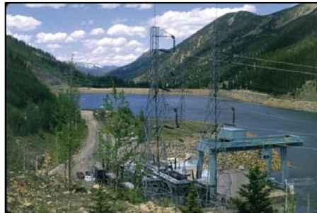
Cabin Creek Station Capacity 300 MW
