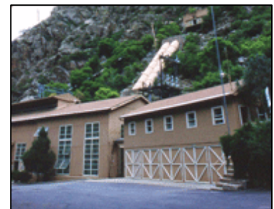
Shoshone Hydro Capacity 15 MW
