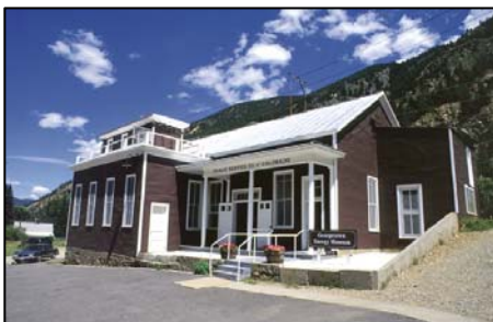
Georgetown Hydro Capacity 1.2 MW
