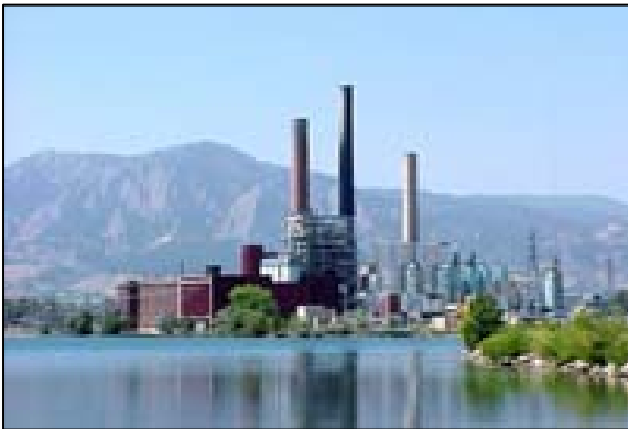
Xcel's Valmont Station near Boulder, Colorado Total Capacity 229 MW: 186 MW Coal-Fired Steam Unit plus 43 MW Gas-Fired Combustion Turbine
