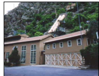
Shoshone Hydro Capacity 15 MW
