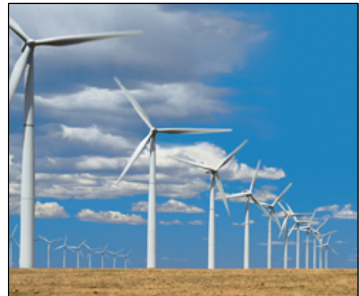
Ponnequin Wind Farm Capacity 30 MW
