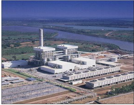
Figure 4. 300 MW National Power Supply plant in Thailand. Two CFBC boilers. Completed Feb. 1999
