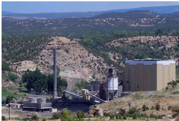
Figure 5. Tri-State's Nucla Station near Nucla, Colorado. One 100 MW CFBC boiler.
