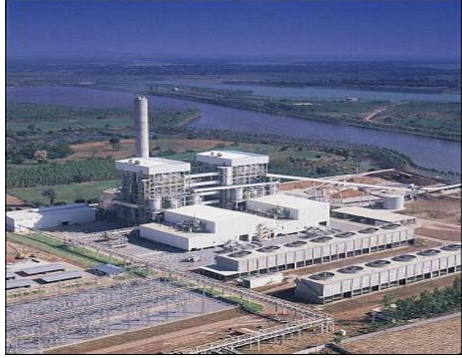
Figure 4. 300 MW National Power Supply plant in Thailand. Two CFBC boilers. Completed Feb. 1999
