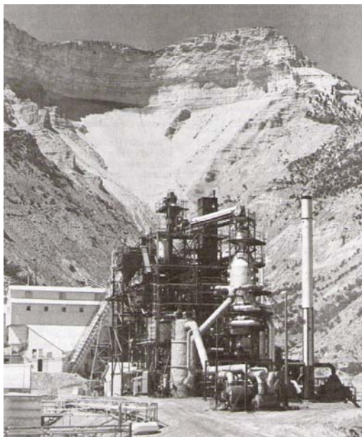
Paraho's 250 t/d Semiworks Unit, Anvil Points, Colorado, ca. 1979
